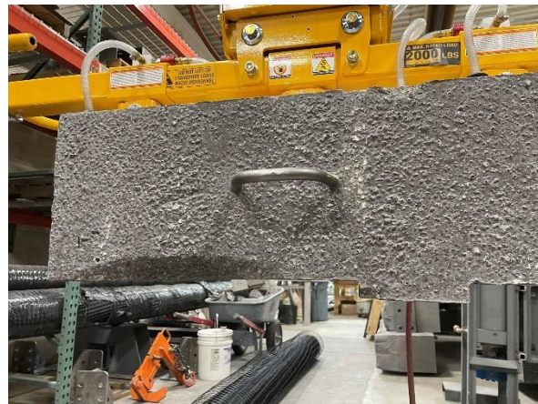
Figure 5 - One shear heel failed, one intact
