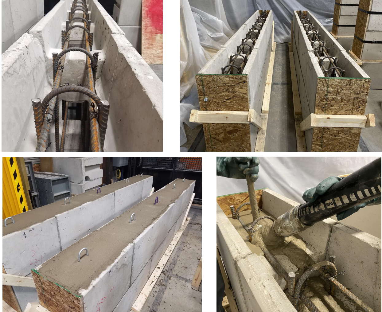
Figure 7 - Construction Photos of Barrier Walls
