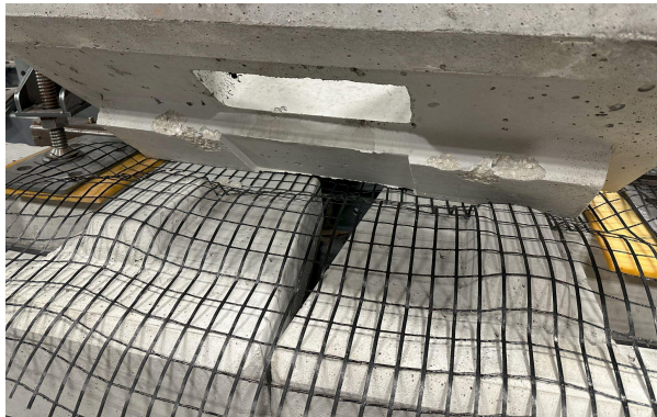
Figure 4 – Groove and slight knob crushing
