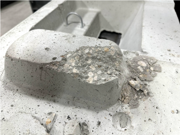
Figure 4 – Broken shear knob
