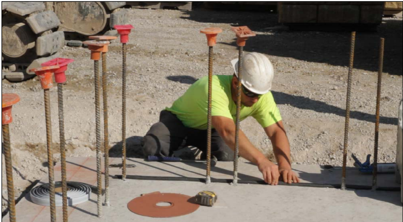
Figure 8: Installing a bentonite/butyl rubber expandable waterstop strip on top of the footing.
