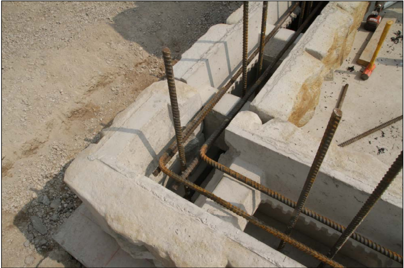
Figure 7: Continuous horizontal rebar through a corner using bars bent 90°. Make sure to follow design standards for minimum development lengths on the bent bars.
