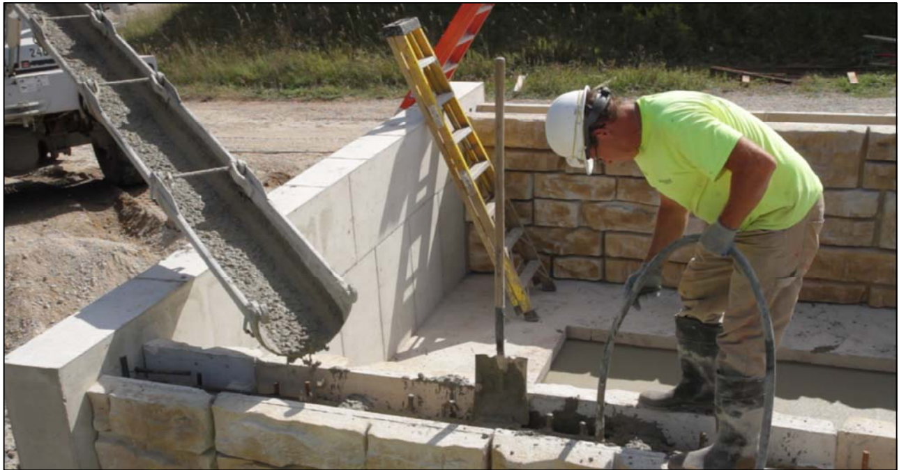
Figure 11: Infilling and vibrating concrete inside the hollow-core wall.
