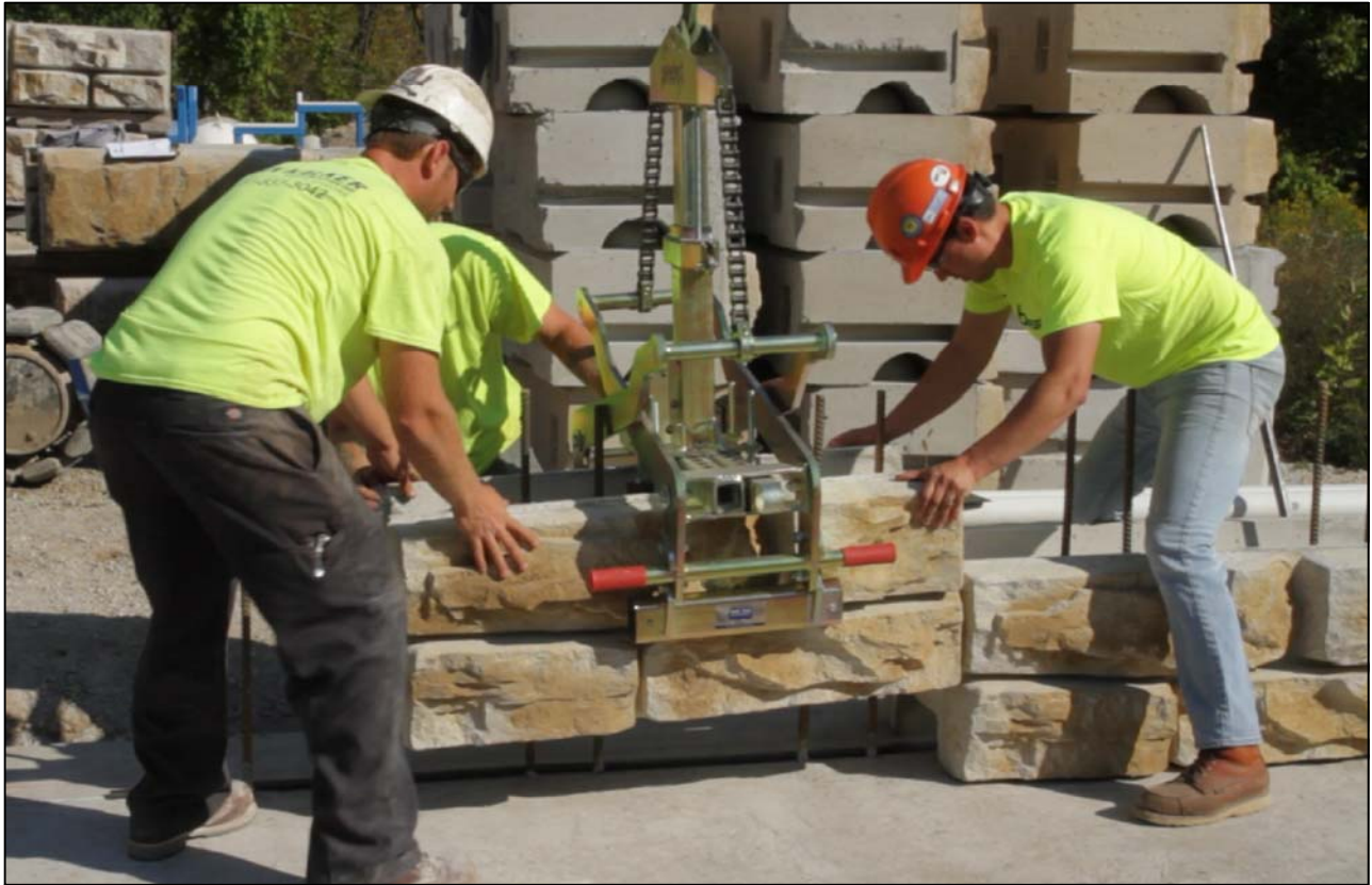
Figure 5: 16 inch clamp requires 17 inch minimum spacing between every other rebar to avoid any conflicts while the blocks are set.
