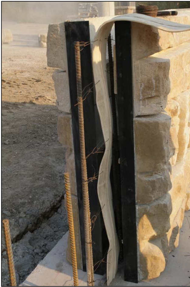
Figure 9: Control joint using ABS plastic along with a PVC ribbed center bulb waterstop secured with wire ties.
