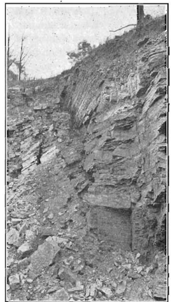
FIG. 3.—CAVING WALL OF OPEN CUT FOLLOWING SLIP PLANES.
