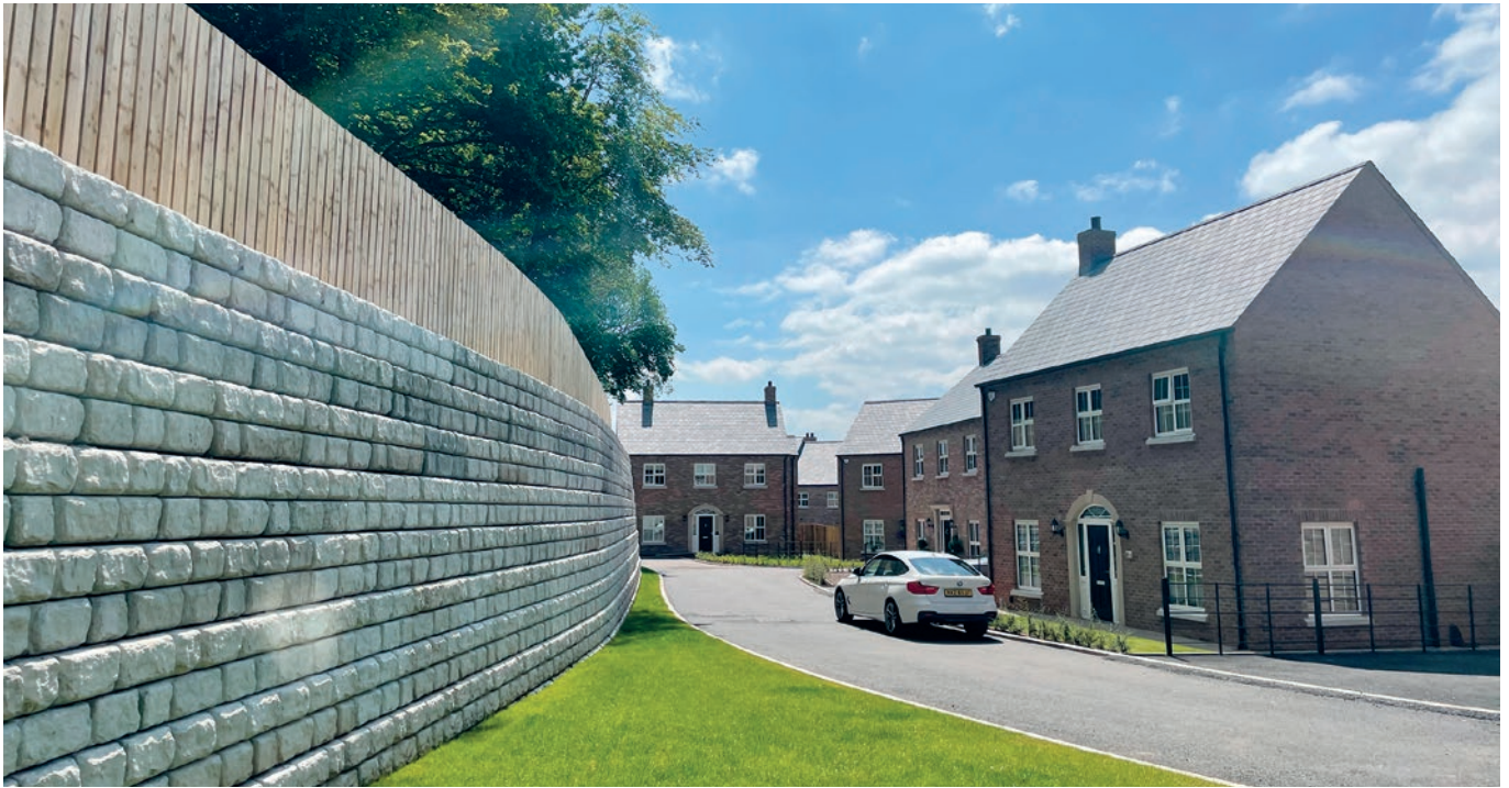
The 280-meter (919-foot) long wall hugged the property line of the development, optimizing the buildable footprint and expediting installation compared to a segmental block retaining wall.
