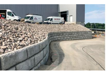
The finished Redi-Rock wall at the COVI meat processing factory in Bressuire winds along the driveway, providing access to vehicles at two levels of the plant.
