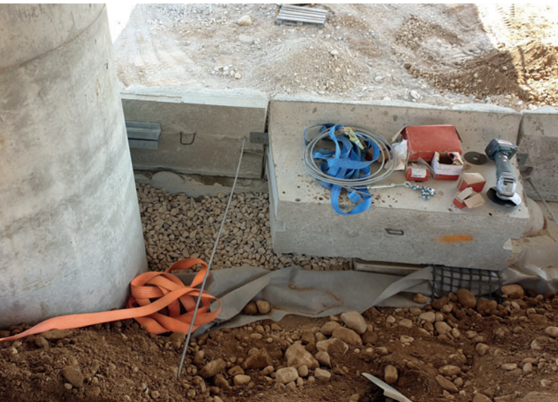
The custom Redi-Rock blocks used to overcome the conflict with the bridge support columns.
