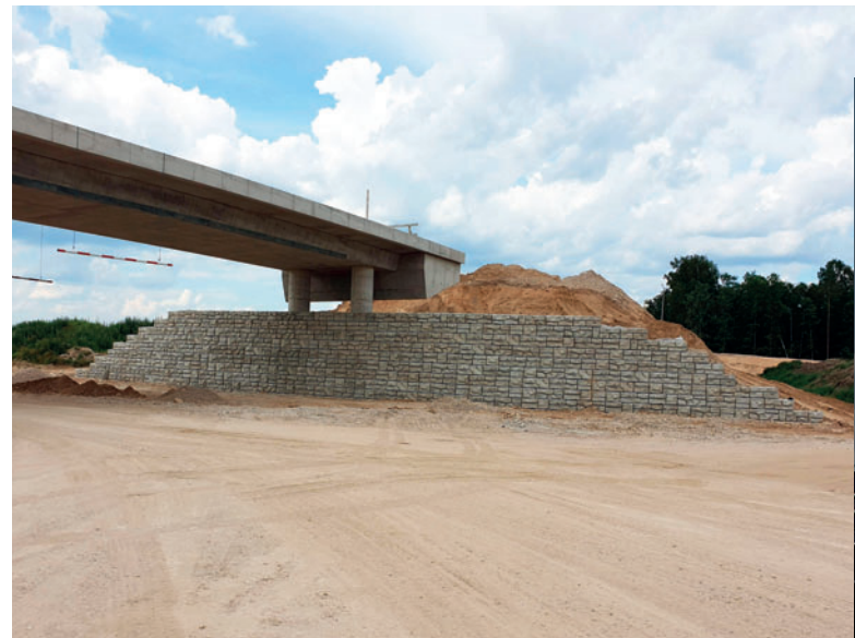
Originally slated to be MSE panel walls, over 600 Redi-Rock PC blocks in the Ledgerstone texture create the wingwalls for the Mustla Bridge.
