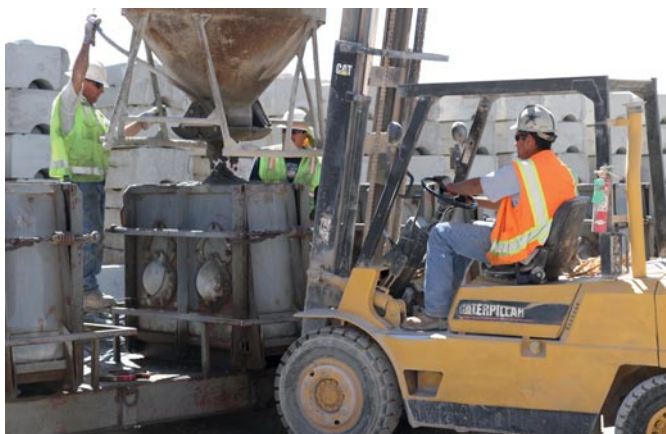
Production of the Precast Modular Blocks (PMB)
