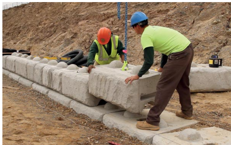
Installation of the PMB on-site
