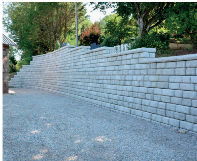
Redi-Rock blocks install like giant Lego blocks using an excavator and small crew.
