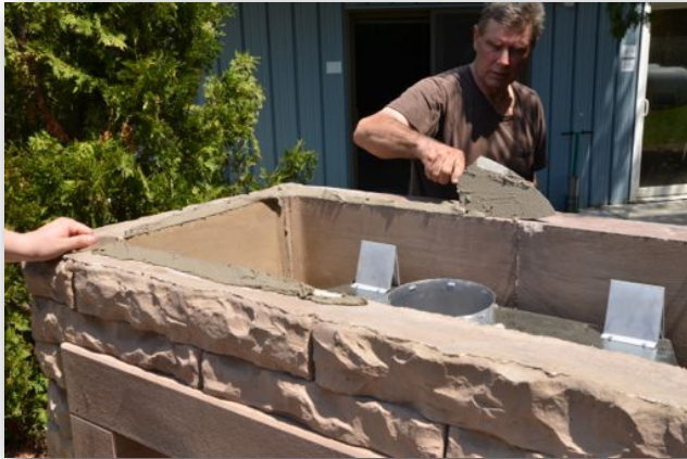
Place mortar on top surface of firebox
