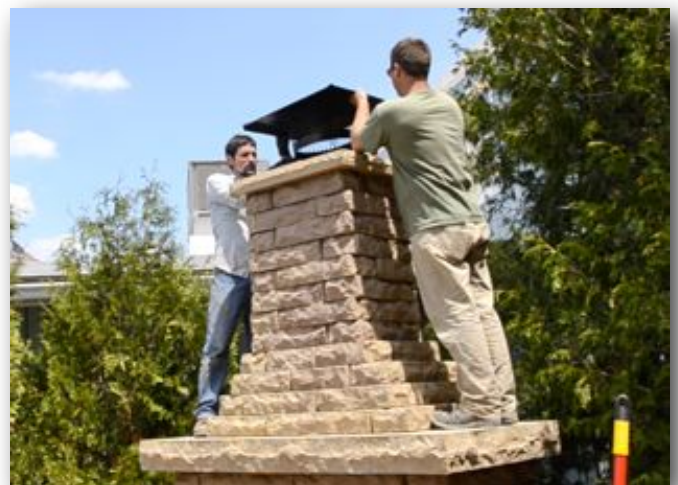
Fasten spark arrestor to outer wall chimney pipe
