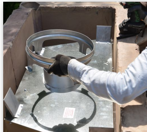
Remove and save the vent collar
