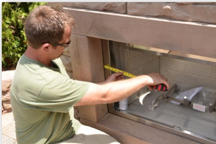
Center and level insert in firebox
