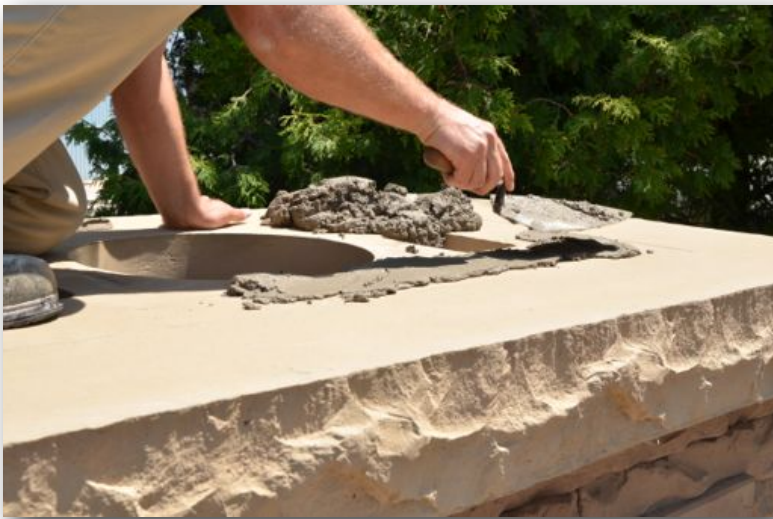
Place a very thin bed of mortar on mantle inside reference lines
