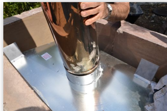
Test-fit inner chimney pipe in opening
