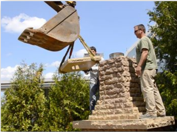
Place chimney cap on chimney with appropriately rated, secured lifting straps
