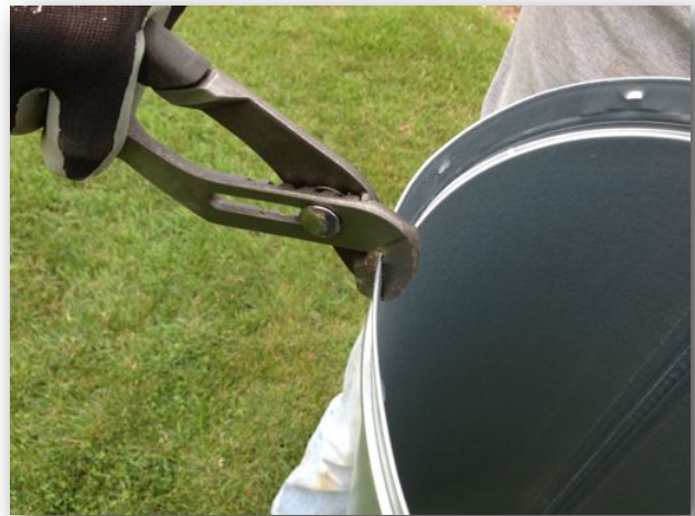
Expand the bottom of outer-wall section
