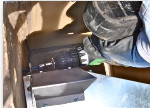
Fasten insert to firebox with screws
