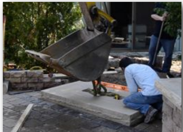
Ensure hearth is level both ways
