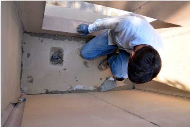
Remove excess mortar and debris
