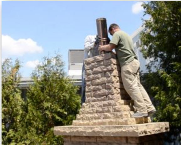
Insert connected inner-wall sections in
