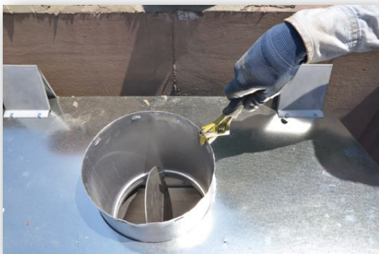
Expand chimney opening
