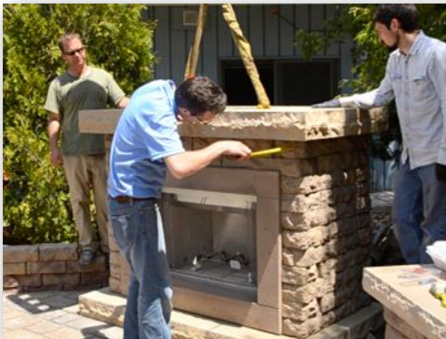
Center the mantle side-to-side (approximate 4.5" overhang), leave a 5" overhang on the front and approximately flush in the back.
