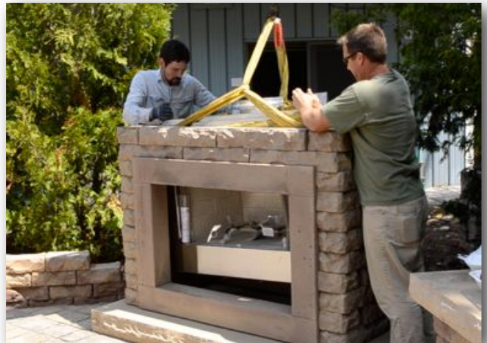
Carefully set insert in firebox.
